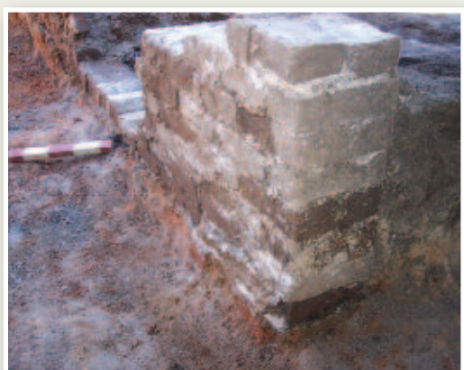
Brick foundation wall
